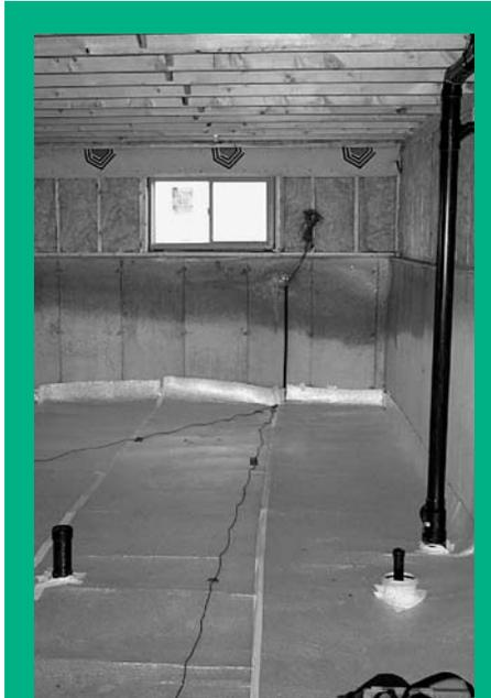
**Bubble-pak insulation scored a rating of just over R-2.**
