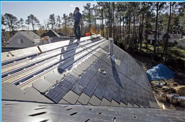
PV shingles. Thin-film PV shingles are designed to blend in with regular asphalt shingles.
