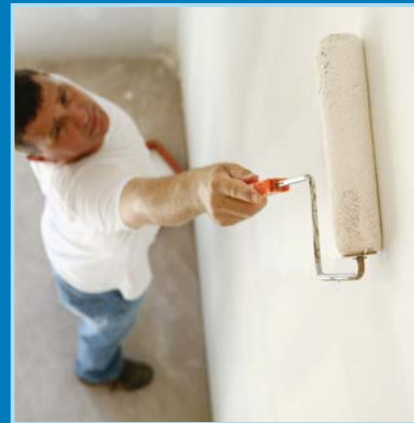
Paint. Low- and no-VOC paints and finishes offgas significantly less than conventional products.
