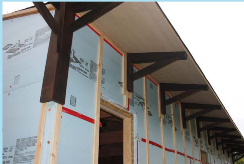
The Hellier home in Bristol, Vermont, is going up green. Among other features, a south-facing orientation (top left and right) capitalizes on natural light and thermal energy, while insulated panels (bottom left) and wrapped framing (bottom right) seal the home. This home also enjoys the advantage of know-how: with experience, builders generally can trim much of the "green premium" from such projects.
