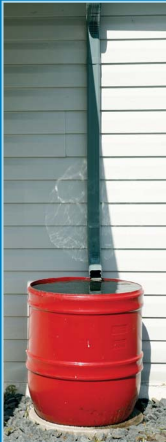
Rainwater collection. Rainwater collected from the roof in barrels or cisterns can be used for irrigation and other nondrinking uses.
